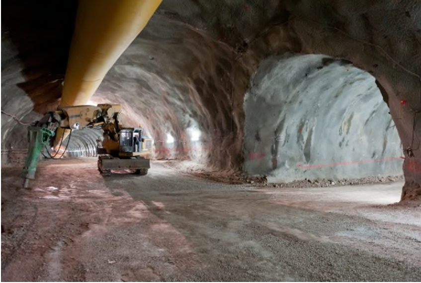
Junction area at Panagopoula T26 Tunnel
